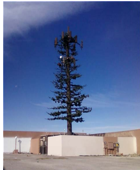
Example of a stealth cellular tower
